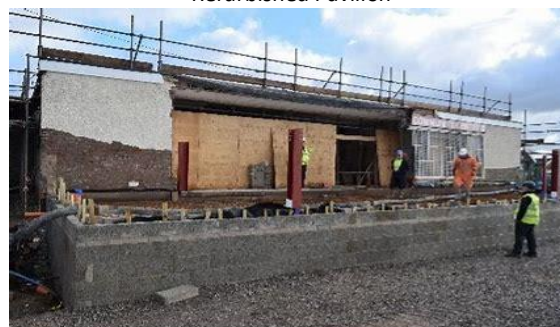
Building Works in progress
